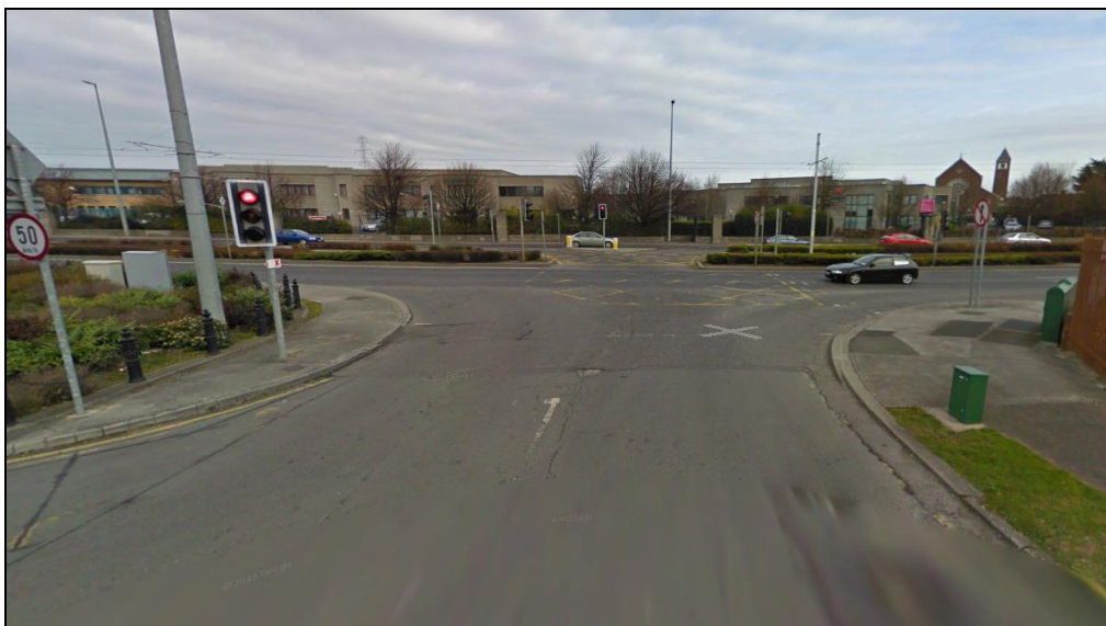
Figure 6.2 - Existing Signalised Junction on the Unnamed Road leading onto the Naas Road.
