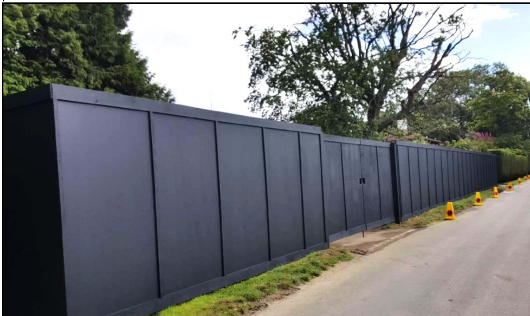
Figure 5.1 – Typical Site Hoarding Arrangement
